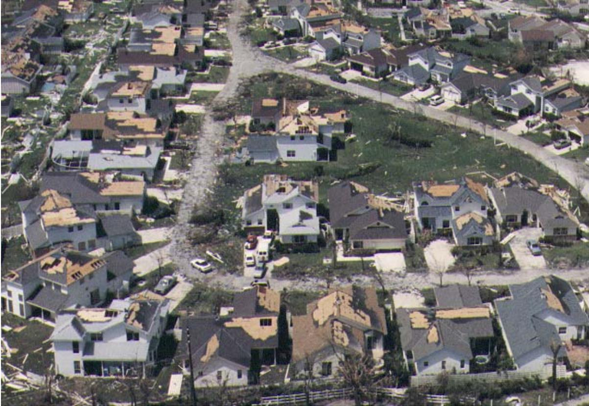
Figure 1. Cladding damage on houses after Hurricane Andrew (1992). Photo courtesy of Applied Research Associates, Raleigh, North Carolina, USA.
