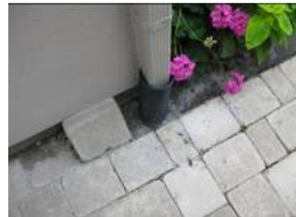
Previous to the retrofit, one downspout drained directly onto the driveway, preventing water from being absorbed by vegetation and causing icing in the winter. A French drain was installed to correct the problem.
