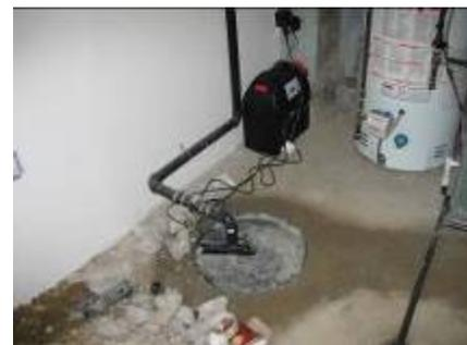
A sump-pump was installed to convey rainwater out of the weeping tiles, bring it to the surface of the lot, and pump it onto the lawn (away from the foundation) in order to keep excess water out of the municipal system.
