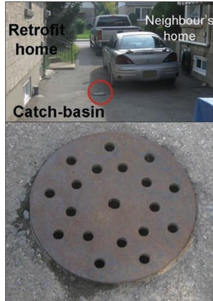
tating installation of additional measures to reduce risk. This catch-basin was connected to the home's foundation drainage; surprisingly, it served to drain the neighbour's driveway, which was sandwiched between the two homes (See Figure 1 above). The catch-basin essentially transformed the neighbour's driveway into a huge funnel that directed massive quantities of rainwater into the foundation drainage and risked overloading of the sump pit and pump during heavy rainfall events.
