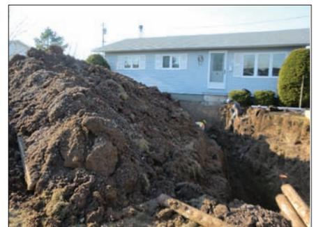
water away from the home quickly; they should never have any standing water. Based on the camera inspection, and before the backwater valves were installed, the laterals had to be torn up and replaced, requiring the excavation of the front yard (See Figure 2).
