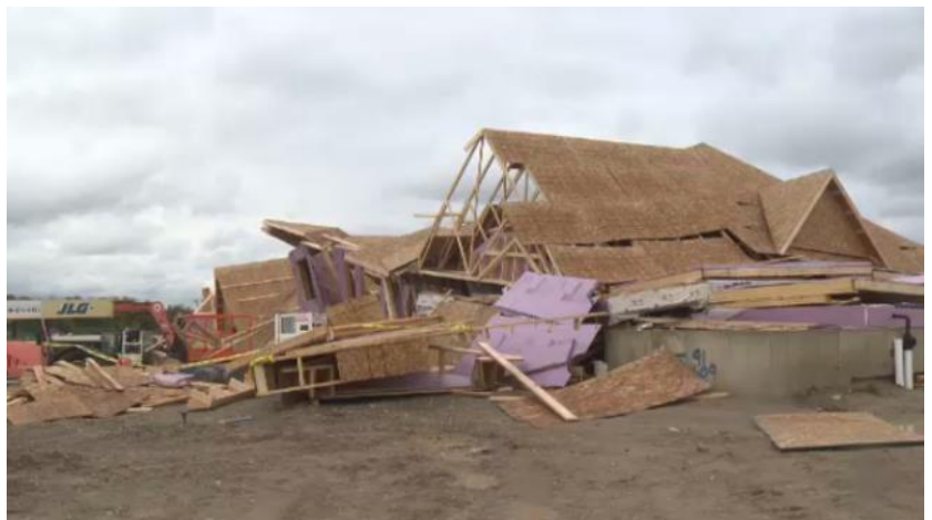
Strong winds lead to the failure of several partially constructed homes in Waterloo, Ontario Sunday, October 15, 2017 (Source: Mike Muncic and CTV News)
