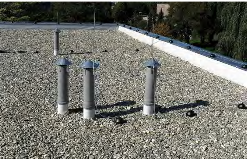
Class A commercial roof.
