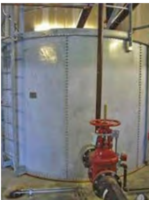
Example of a 60,000 litre (15,000 gallon) steel secondary water supply tank. Tanks such as these are commonly anchored to the floor to prevent them from sliding or tipping during an earthquake.
