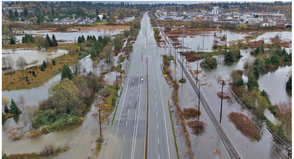
Flooding on B.C. Highway 11 in November 2021. Photo: BC Ministry of Transportation and Infrastructure/Flickr.
