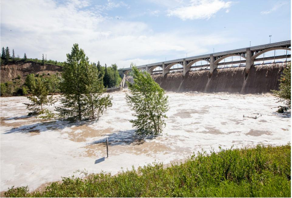
**Figure 20:** *The Glenmore Dam overtopped during the 2013 flood but remained invaluable as its operation reduced peak downstream flow. (Source: City of Calgary)*
