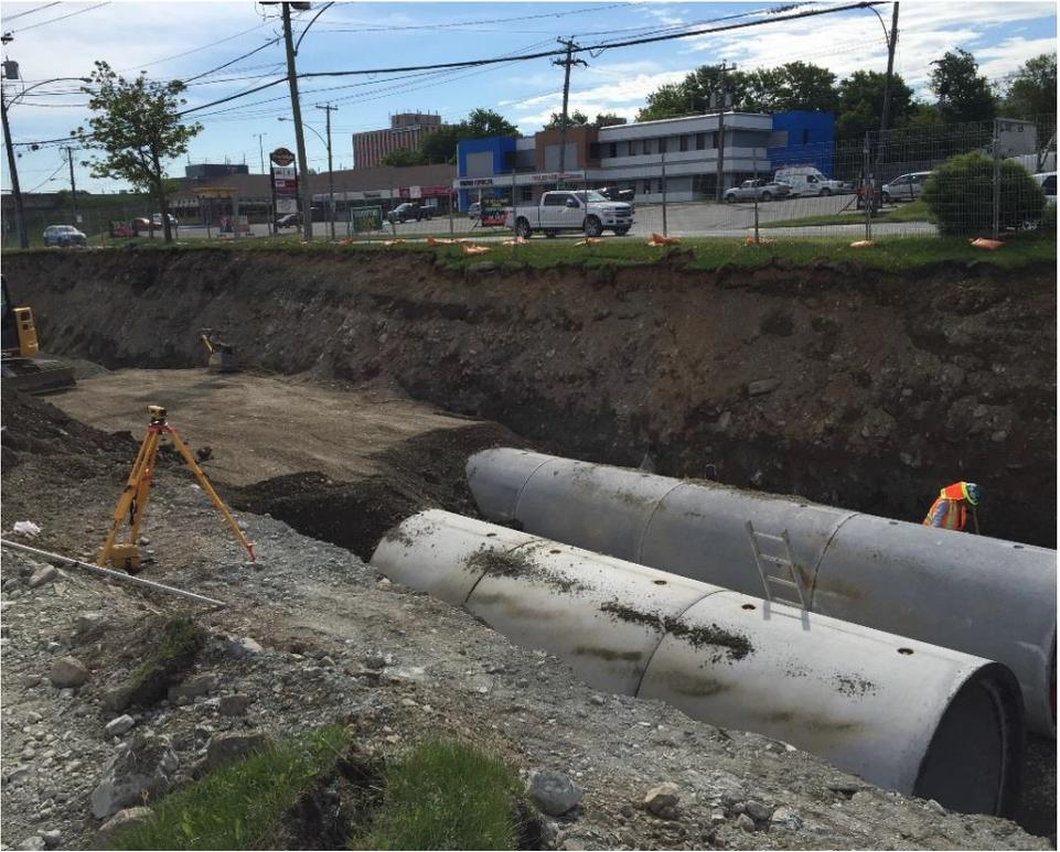
**Figure 19:** The new sewer ranges in size from 200% to 400% greater than the previous pipes that were in place. (Source: City of St John's)
