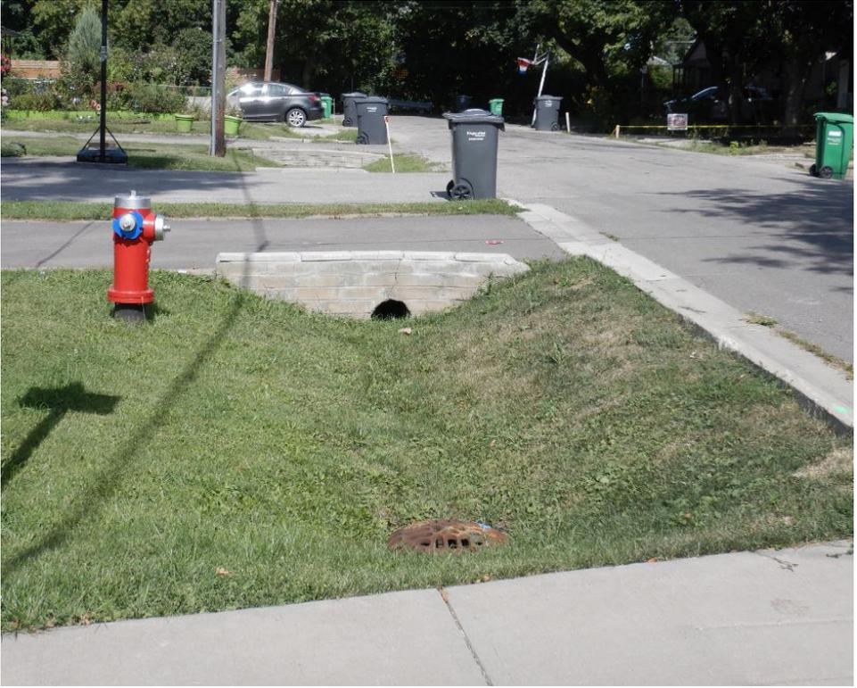
**Figure 16:** City of Mississauga low-impact development feature located on First Street. The LID is composed of both bioswales and permeable pavements. (Source: City of Mississauga)
