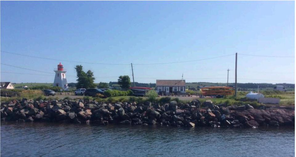
**Figure 11:** *Victoria-by-the-Sea rebuilt its seawall using large granite boulders.*
