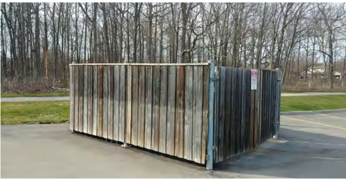
Garbage containment areas should be built with non-flammable materials and be located at least 10m from the building.
