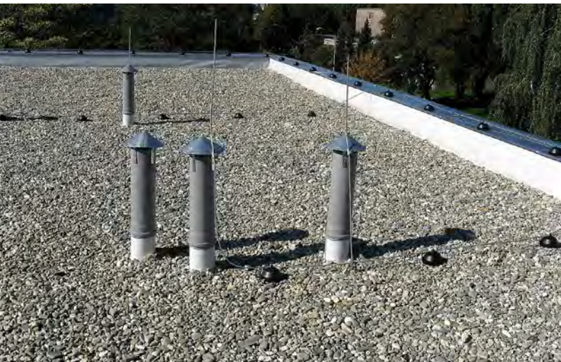
Class A commercial roof.
