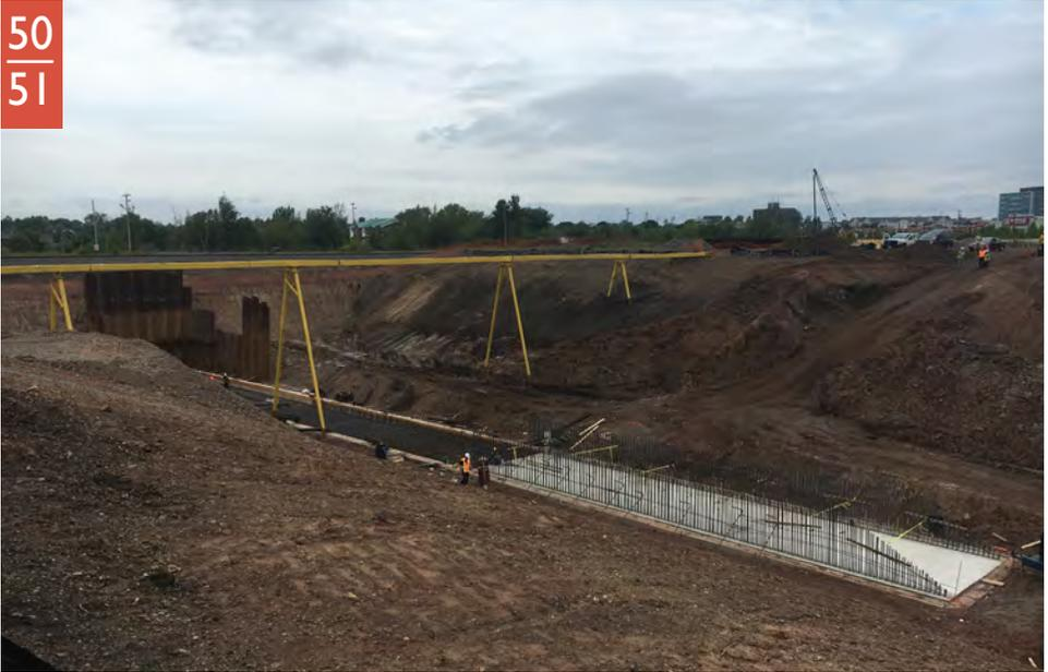
**Figure 12:** Construction of the new culvert in Moncton.
