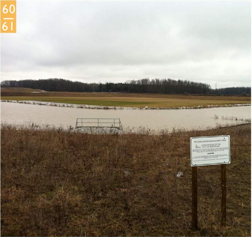
**Figure 16 :** Stormwater management pond built in Stratford to accommodate surcharging of local systems.
