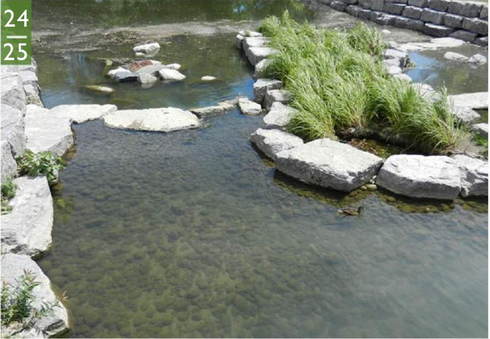
**Figure 6 :** *The Victoria Park Lake Improvement project includes a new sediment forebay. It is designed as an initial storage area to trap and settle out sediment and heavy pollutants before they reach the main basin. (Source: ICLR)*
