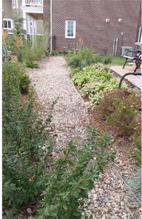
**Figure 25 :** The pictures above show an infiltration trench built in the Currie Barracks Brownfield re-development project. An infiltration trench is an excavated trench backfilled with stones to create a narrow underground reservoir. Stormwater runoff diverted into the trench drains from the bottom of the trench into the subsoil and eventually to the water table.
